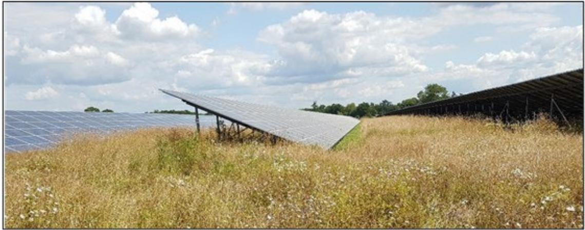
Figure 4.3: Sites where a “Shade Cut” has been employed during the growing season to prevent shading of panels, but allow flowering meadow elsewhere
